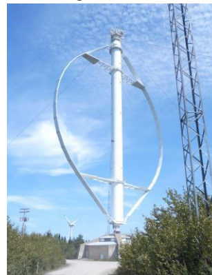
Fig. 4: Vertical-axis wind turbine – Darrieus-type. Source: Wikipedia, 2018.
